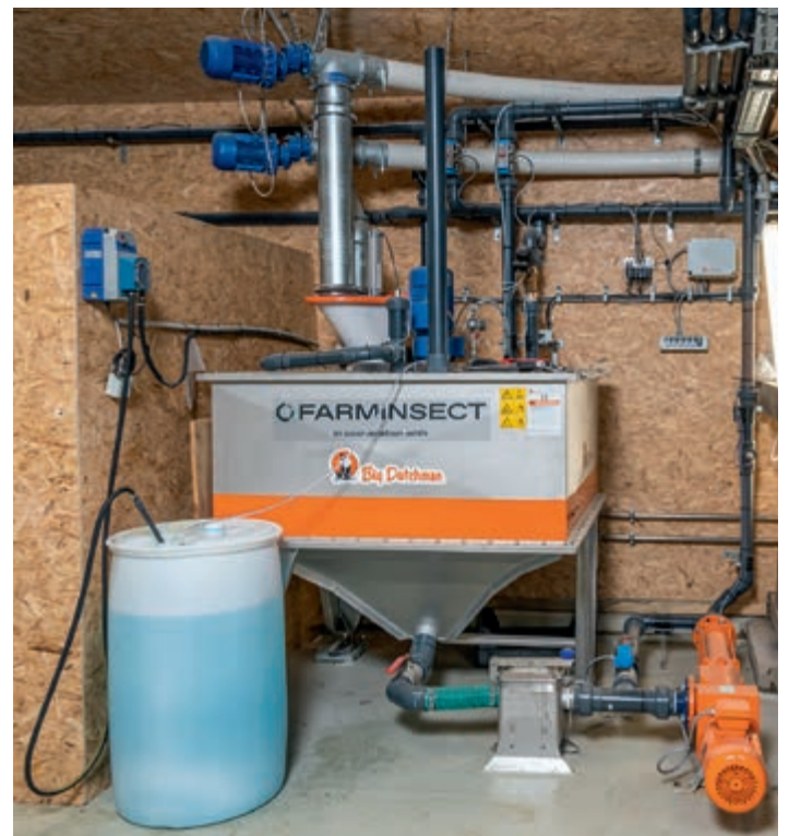
The feed mash is mixed in two mixing tanks, controlled by a computer. Both mixing tanks are placed on load cells for this purpose
